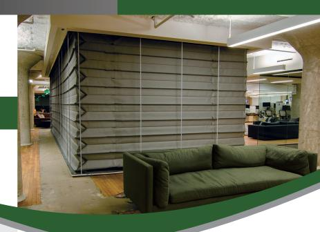
Codes and Standards. M4000 fulfills IBC requirements to provide an opening protective where these assemblies are permitted as passive barriers used smoke control systems. This fire-rated curtain system can serve as opening protective in applications such as an atrium, stairwell and escalator construction.
